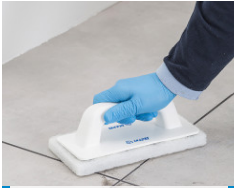
Removing traces of product visible after a few hours with a Scotch-Brite® pad
