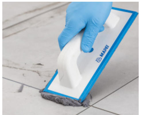
Grouting the joints with Flexcolor 4 LVT
