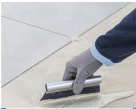
Spreading Ultrabond Eco 4 LVT and bonding LVT tiles with wide joints and spacers
