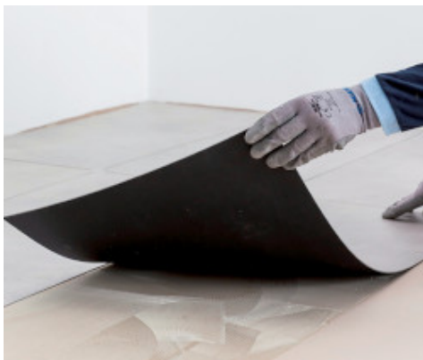
Bonding LVT tiles with Ultrabond Eco 4 LVT
