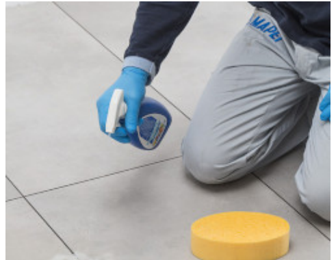
Final cleaning operation with Kerapoxy Cleaner
