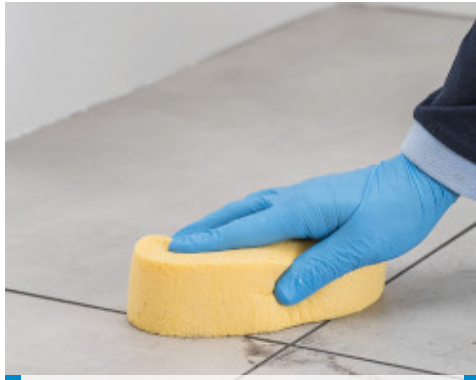
Removing traces of Flexcolor 4 LVT with a sponge from the surface of the tiles
